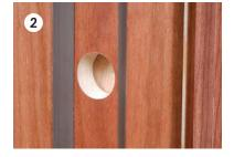
The striker installation has never been so simple: it just takes a milling of  $\emptyset$  25 mm and a drill. Jigs are not required.
