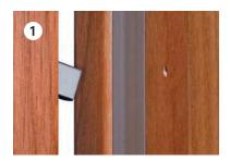
After the installation of the lock and the throw of the hook, by softly pushing the door against the jamb it is possible to centre the striker.
