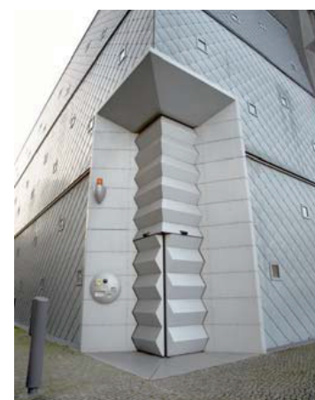
Cornered automatic door
