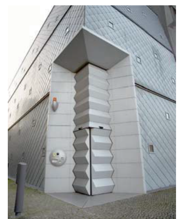
Cornered automatic door
